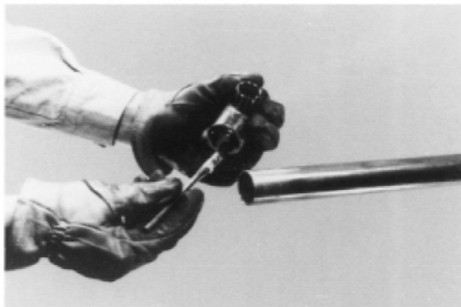
FIG. 11 Fluxing: Fitting
